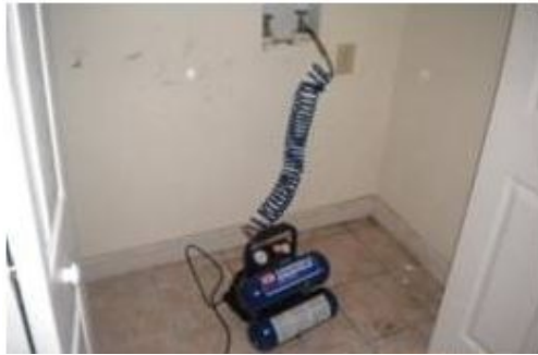
Water blown out of Lines
