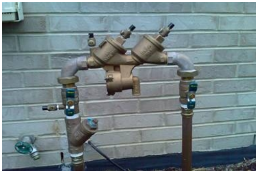
Radiant Winterization RPZ Valve
